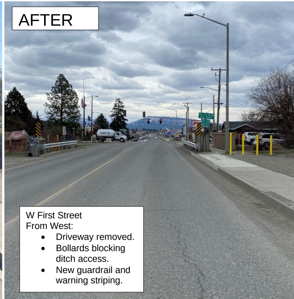
FIGURE 3 – 2021 CAPITAL IMPROVEMENTS – 1 ST STREET GUARDRAIL, SIGNS, AND ACCESS CONTROL
