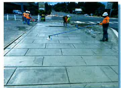
First Street Storm Drain and Billings Avenue Intersection Improvements
