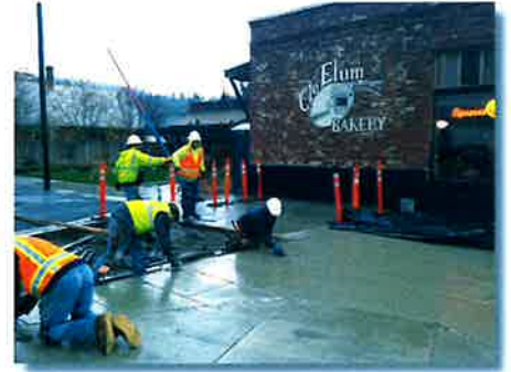
SR 903 and Peoh Avenue Improvements
