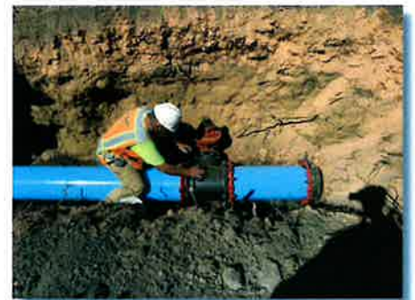
SR 903 Utility Extensions
