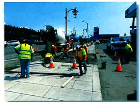
First Street Downtown Revitalization Phase 3A
