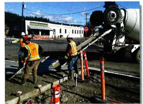
SR 903 and Peoh Avenue Improvements
