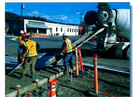
SR 903 and Peoh Avenue Improvements
