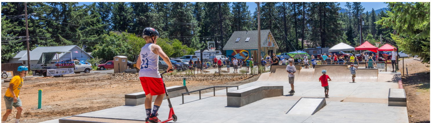
Open area where Phase 2 will be constructed is on the left. Currently, user flow is constricted because of the narrow width, which will be resolved once the skatepark is completed.
