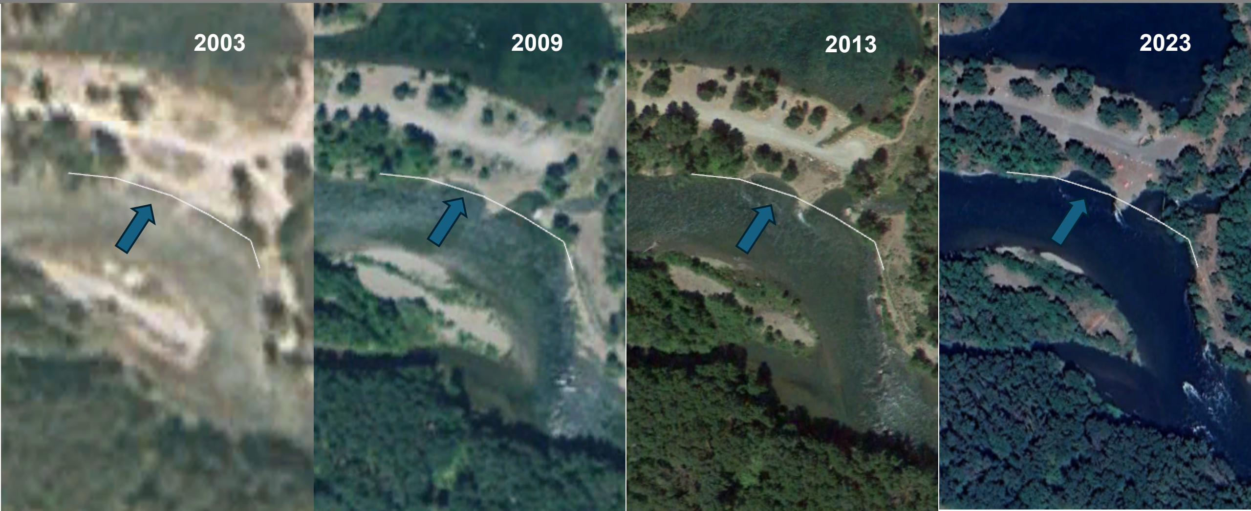
Progression of continued bank erosion
