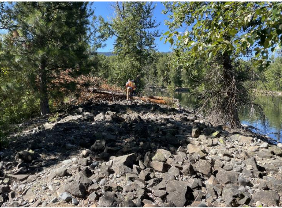
PHOTO 5: Embankment erosion near parking area from Yakima River flows. Photo viewing east.
