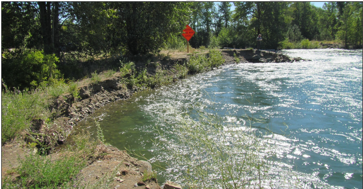
Figure 3. Photo of the eroding bank of concern with riprap spur visible at the downstream end of the bank (a person standing on spur). (Photo: 8/7/ 2020).
