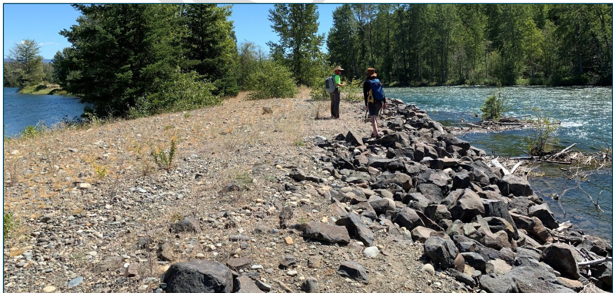
Figure 9. Riprap reinforced levee at RM 186.51. Middle Hanson Pond on the left side of the levee and mainstem Yakima River on the right side – 8/7/2020.
