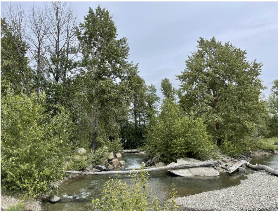
Photograph 2. Side channel to mainstem Yakima River where proposed mainstem channel would be relocated and Option A would outfall. Existing outfall pipe runs under this channel.
