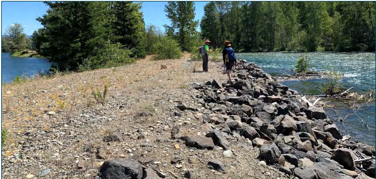
Figure 7. Riprap reinforced levee at RM 186.51. Middle Hanson Pond on the left side of the levee and mainstem Yakima River on the right side – 8/7/2020.
