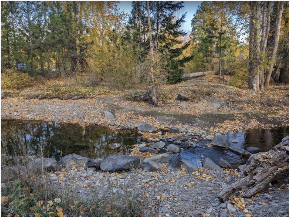
PHOTO 4: Spill channel constructed in 2004 to allow a fraction of flow from the Yakima River to enter the Upper Pond. Photo viewing east.
